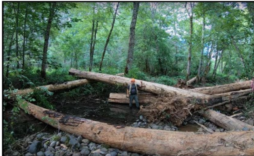
← Large woody debris being placed in key locations in reactivated side channels.
